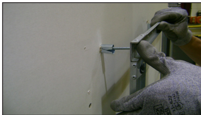
Figure 4.11 Installing Anchors in Hollow Wall
