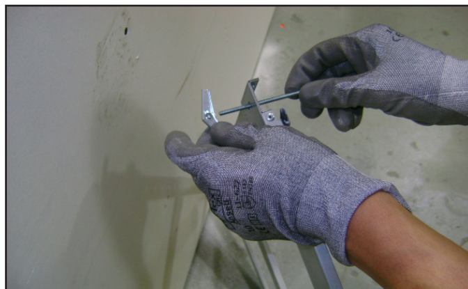
Figure 4.10 Toggle Bolt Installation through Mounting Bracket
